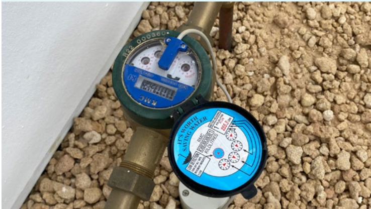
Water meters with electronic monitoring
