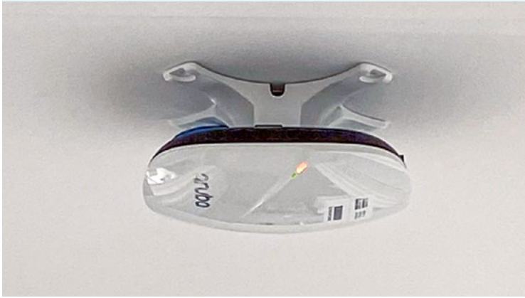
Wireless access point to provide commercial grade internet connection
