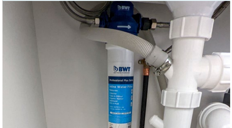
WFA HiFlow inline water filter system
